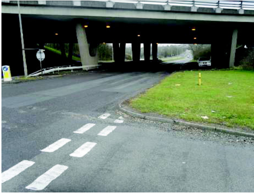
Photo 5 – Shadows formed beneath the M11 over bridge may make it difficult to identify approaching motorists.
