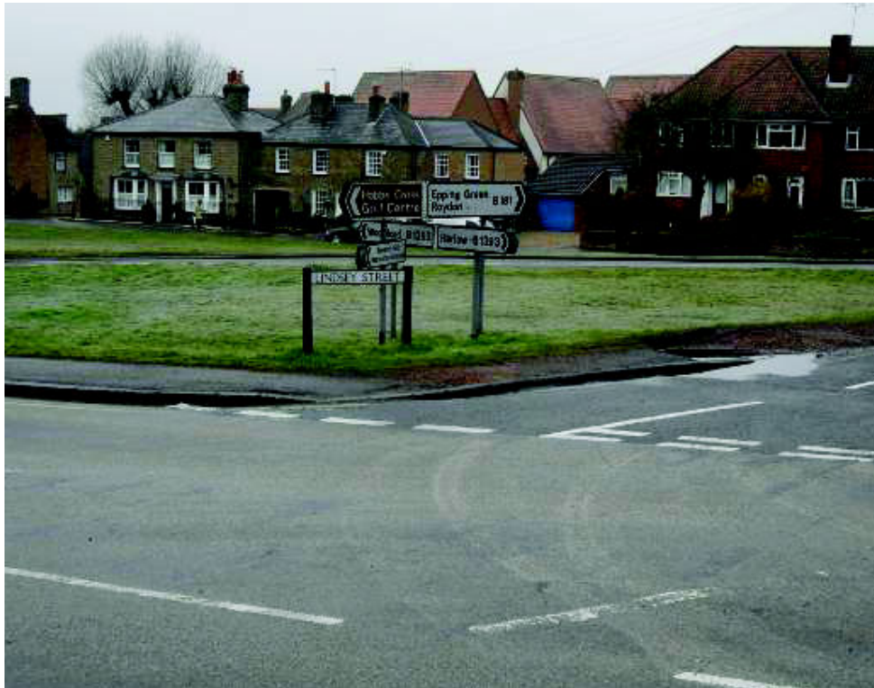
Photo 6 – Numerous traffic signs resulting in sign clutter on corner of the junction.
