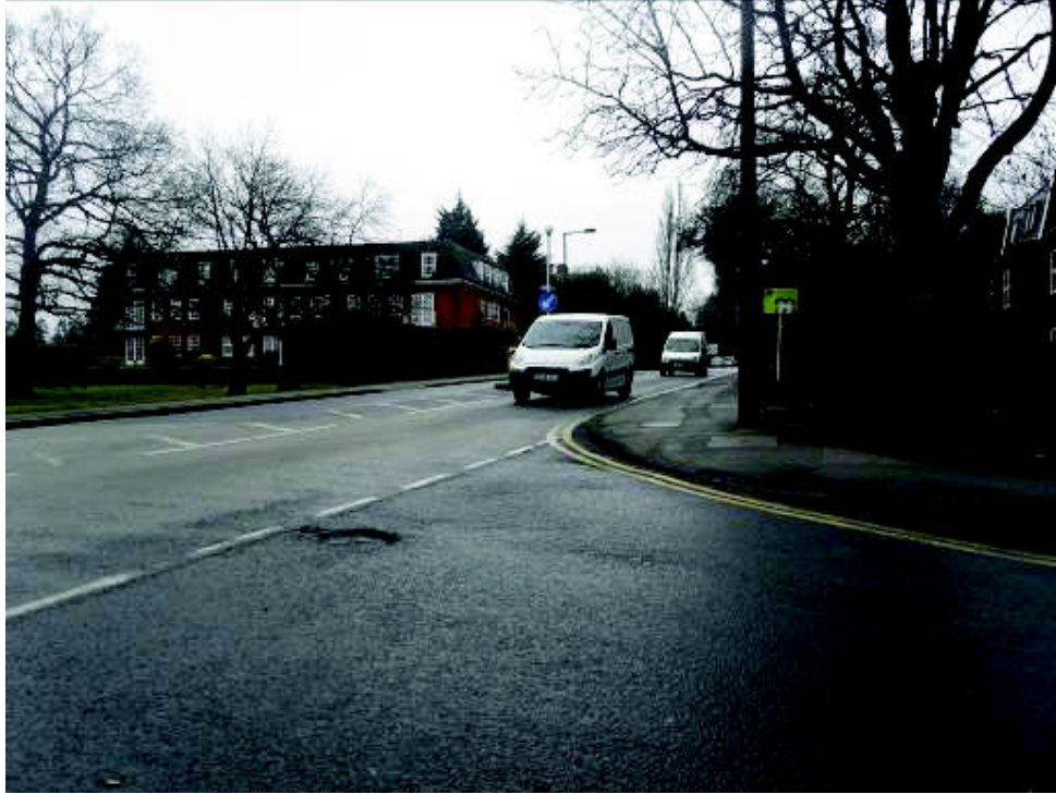
Photo 1 – Visibility splay impeded by street lighting column and overgrown hedge.
