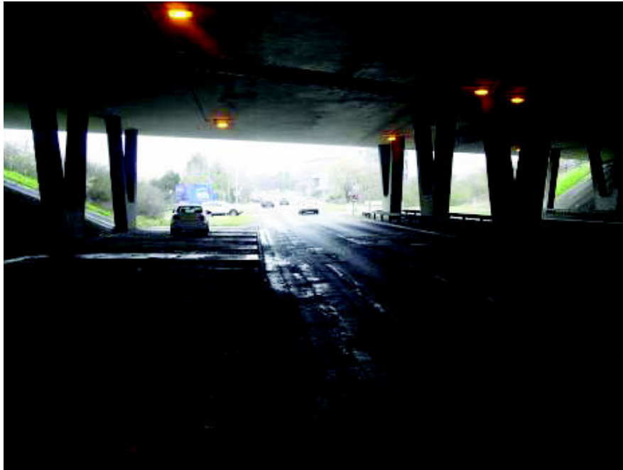
Photo 6 - Shadows formed beneath the M11 over bridge may make it difficult to identify vehicles turning across the path of north-west bound motorists.
