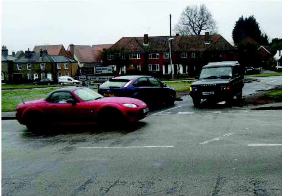
Photo 5 – Kerb being over run as the link road is not wide enough for two opposing vehicles.
