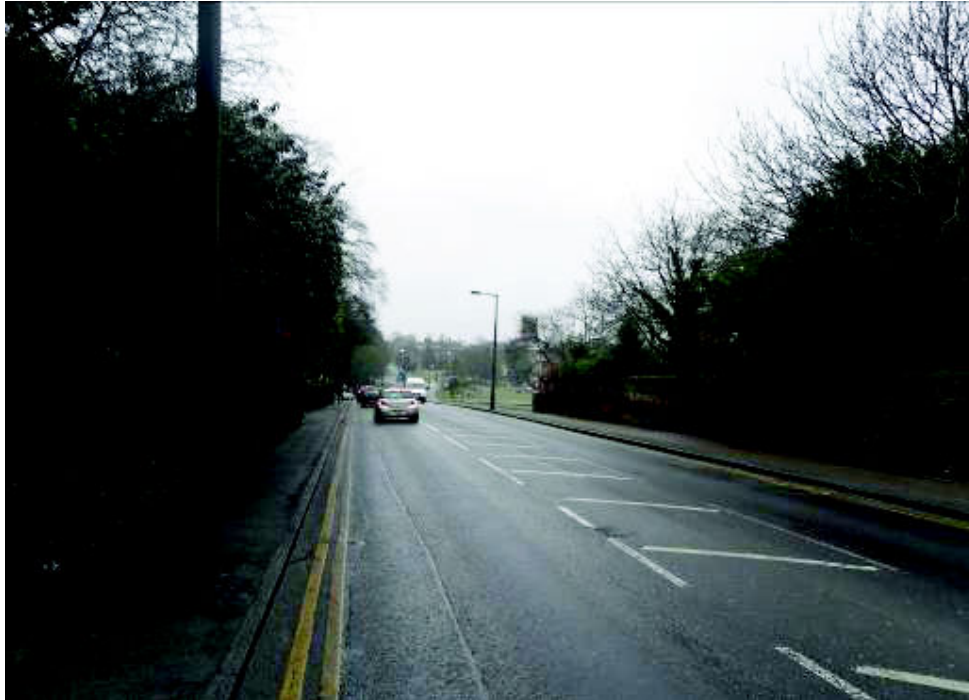
Photo 3 – Misleading 'Staggered junction ahead' warning sign partially obscured by overgrown vegetation.
