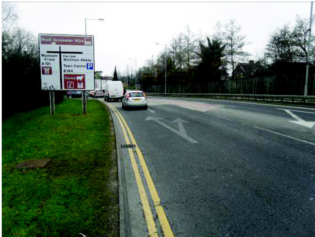
Photo 4 – Advanced directional sign on A121 Meridian Way northbound approach. Also shows worn directional arrow markings.
